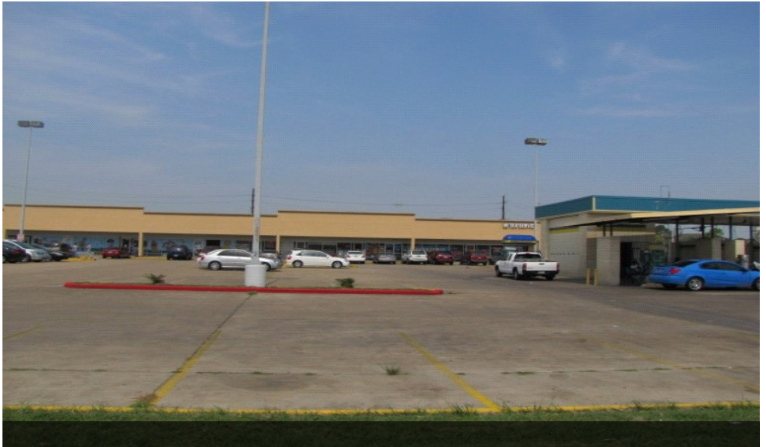
Parking other view
